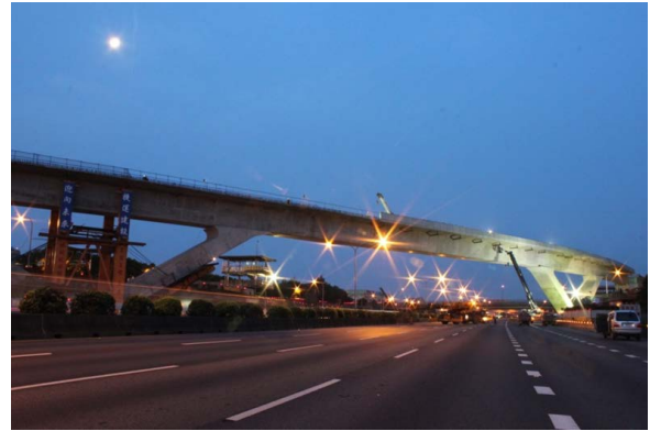
Figure 18. The real photo of CE02 V-type bridge after constructed 图 18. CE02 V 型桥完工后实景
