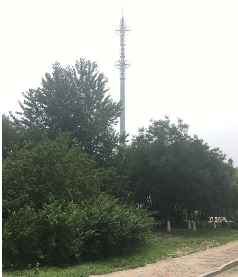
Figure 5. Tower photograph 图 5. 铁塔实物照片
