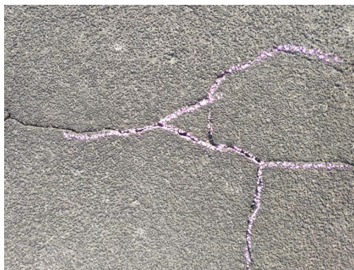
Figure 2. Crack to be measured 图 2. 待测裂缝
