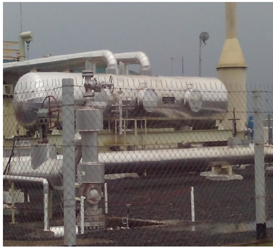
Figure 2. The horizontal water/steam separator 图 2. 卧式汽水分离器
