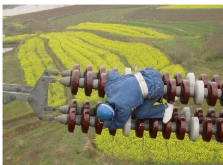
Figure 1. Cleaning insulators
