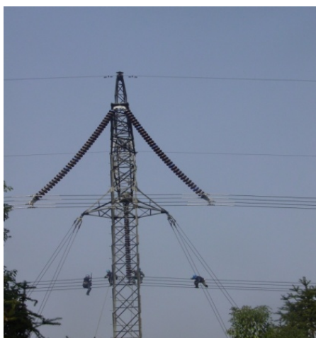
Figure 2. V shape insulator string 图 2. V型绝缘子串
