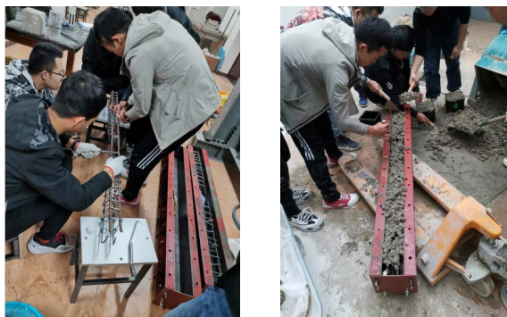
Figure 3. Fabrication and pouring process of reinforcement skeleton
