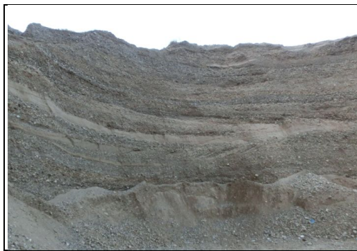
Figure 13. The diagram of the exploitation surface of recently deposited sand and cobble stratum
