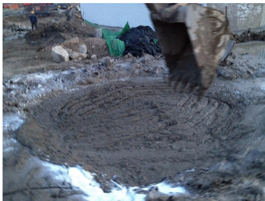
Figure 10. The effect of add lime after stirring in 2# pool
