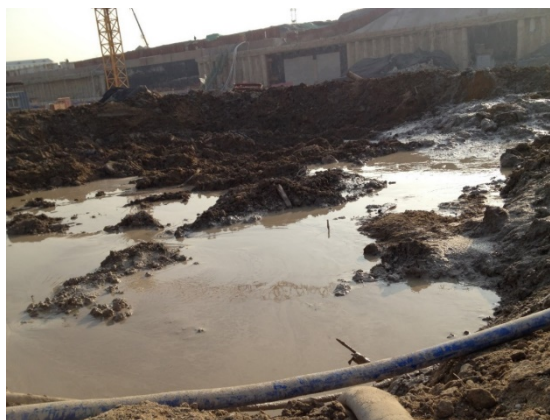
Figure 1. Picture of waste slurry on the construction site 图 1. 施工现场废弃泥浆图
