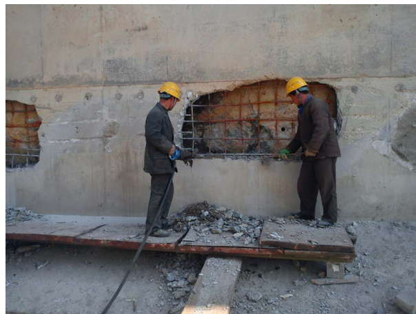
Figure 5. Removal of damaged concrete in site
