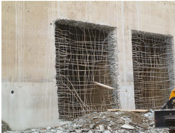
Figure 6. Rebar reposition at damaged spots
