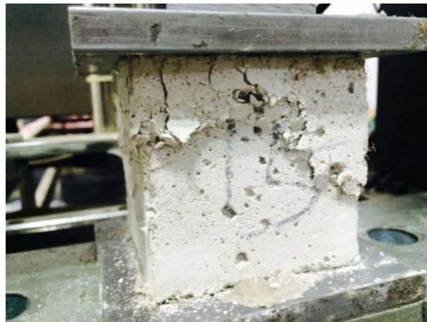
Figure 4. Well versed inclined cracks 图 4. 贯通的斜裂缝
