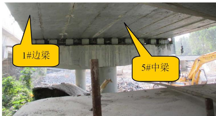
Figure 1. The location of the beam for destructive test
