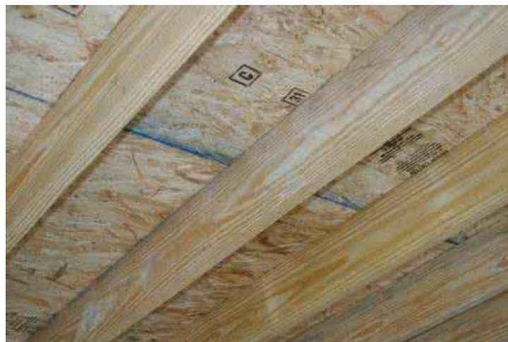
Figure 2. Joist made of saw lumber 图 2. 实木搁栅
