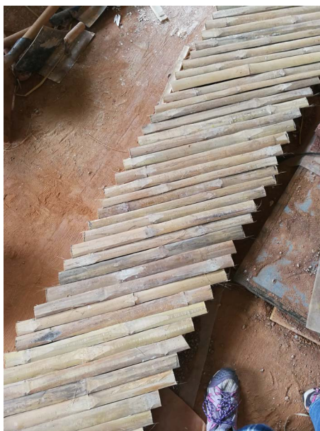
Figure 7. Bamboo strips nailed on skeleton 图 7. 骨架上安装好的竹片
