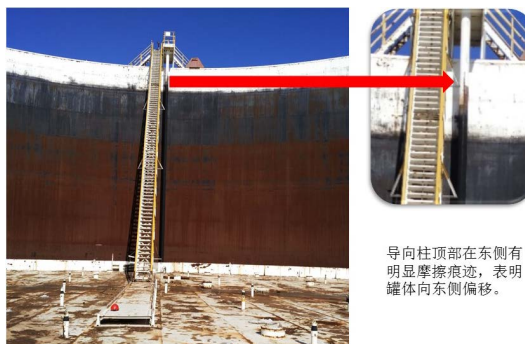
Figure 7. Internal state of storage tank 图 7. 储罐内部状态照片
