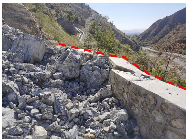
**Figure 3.** Damage from rain-induced landslides
