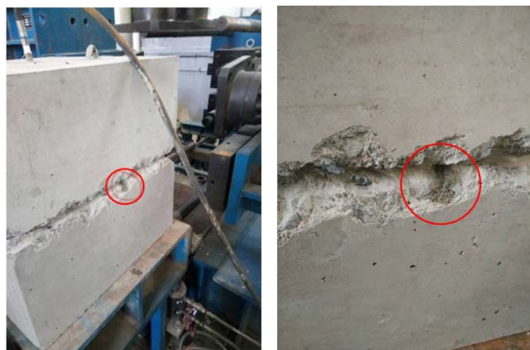
Figure 5. The water seepage of component with W type waterproof product of bending angle 30° 图 5. 弯折 30°的 W 型部材试样渗水
