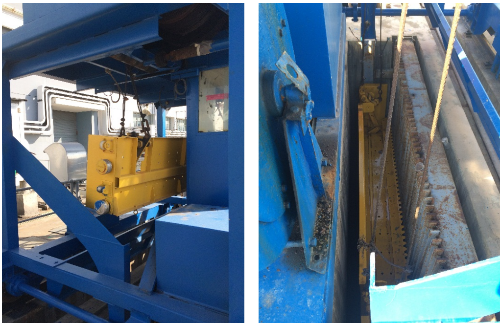
Figure 1. Appearance of the clean system 图 1. 华能玉环电厂拦污栅清污机外观
