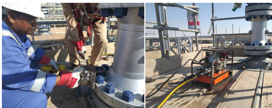
Figure 4. Tightening the bolts 图 4. 螺栓紧固施工
