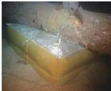
Figure 10. Physical picture of grouting bag method
