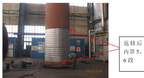
Figure 5. The finished work of repairing the inner cover
