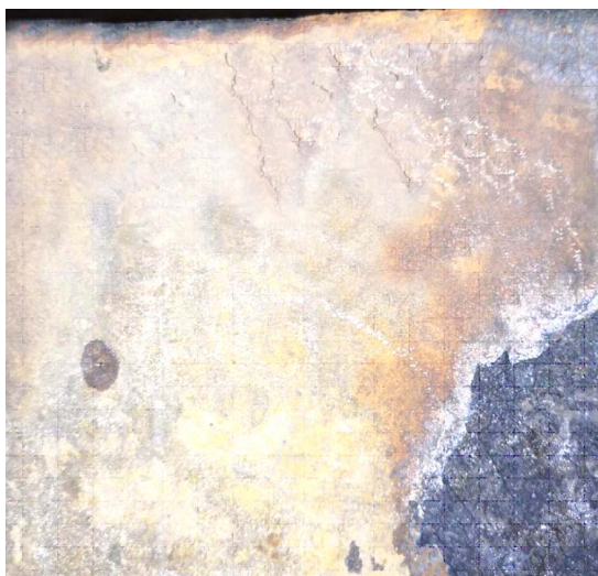
Figure 9. Macro morphology of cracks on longitudinal Plane of 300 mm slab
