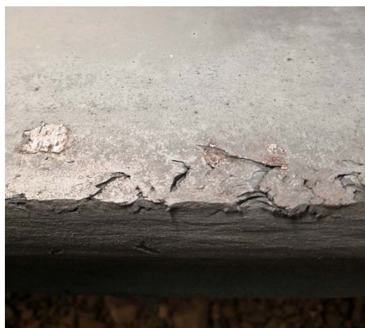
Figure 1. Morphology of edge defect of 60 mm thickness 45# plate
