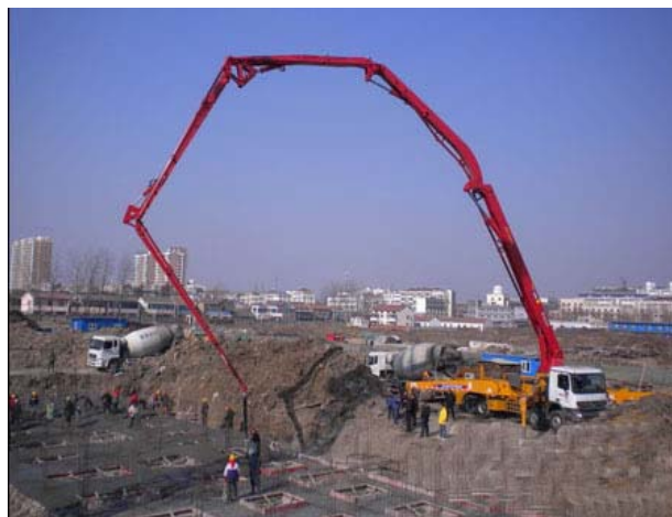
Figure 1. Concrete pump's working situation 图 1. 混凝土泵车工作情景
