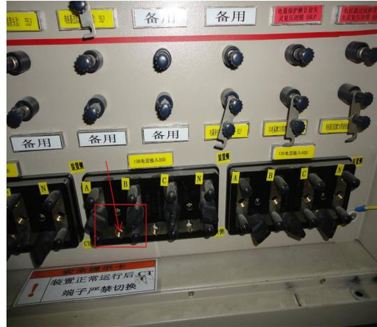
Figure 4. short circuit of A phase and B phase of 13B current terminals
