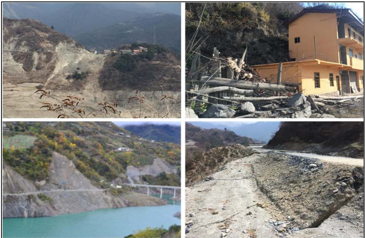
Figure 4. Damaged roads and houses along the vicinity of the Qiao Qi reservoir 图 4. 硃碛水库周边公路、房屋因滑坡受损情况
