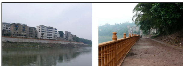
Figure 4. Rentuo landslide after management landscape 图 4. 仁沱滑坡治理后景观
