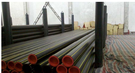
Figure 3. Had the knock against measures for material storage 图 3. 材料的存放要有防磕碰措施
