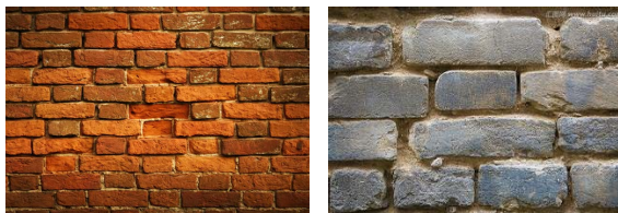
Figure 1. Old brick wall and its mortar joints 图 1. 老旧砖墙及其灰缝
