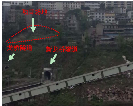
Figure 1. Position relationship between the tunnel and project site 图 1. 既有隧道与项目场地位置关系
