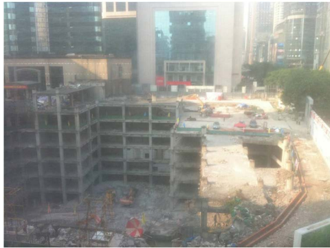
Figure 1. Unfinished building foundation pit 图 1. 原万豪酒店二期烂尾楼基坑
