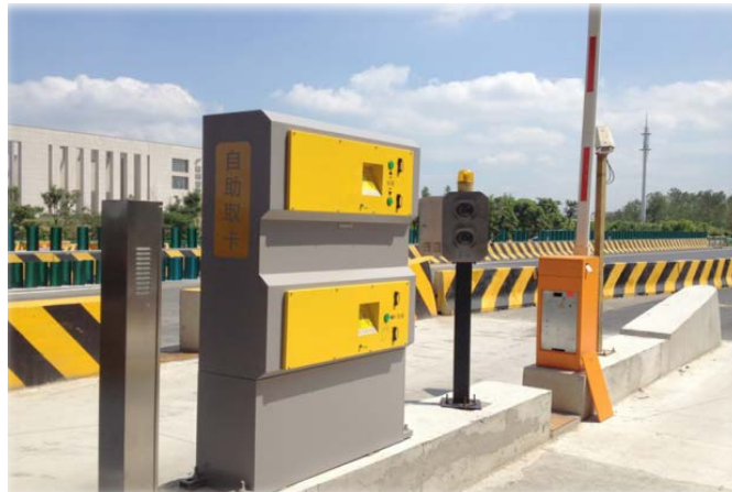
Figure 5. The card machine applied in Hujia expressway overhaul project
