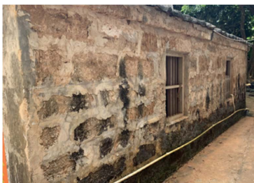
Figure 3. Coral brick wall 图 3. 珊瑚石砖墙
