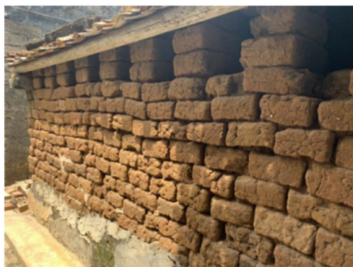
Figure 4. Yellow adobe brick wall 图 4. 黄土坯砖墙
