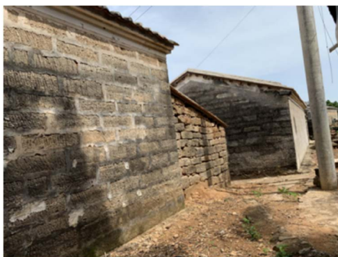
Figure 2. Crater stone brick wall 图 2. 火山石砖墙
