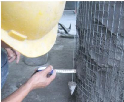
**Figure 5.** Production of steel pipe column protective layer cake
