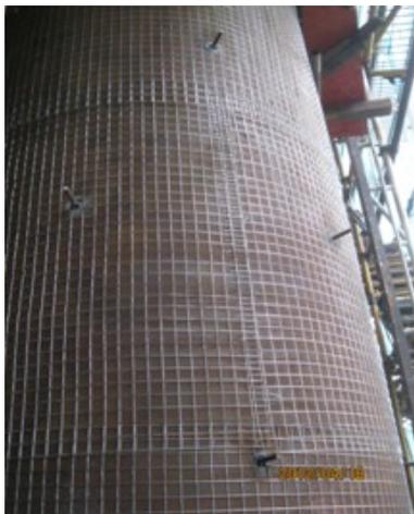
Figure 4. Hanging the first wire mesh
