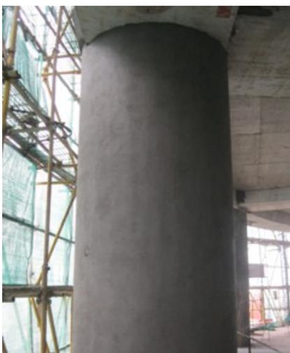
**Figure 6.** Protection of steel pipe column (keep moist)
