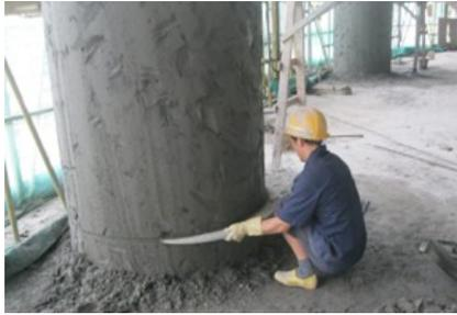
**Figure 7.** During the process of self inspection and control of circular arc mold
