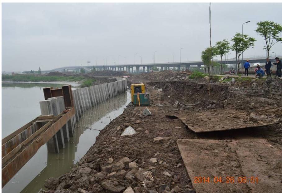
Figure 2. Field photos of U type sheet pile inclined section
