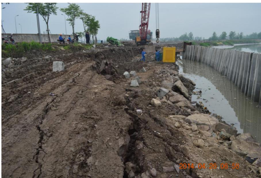
Figure 3. Field photos of U type sheet pile inclined section
