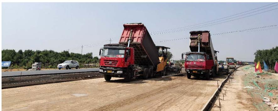
**Figure 1.** Site construction drawing of cement stabilized macadam base
