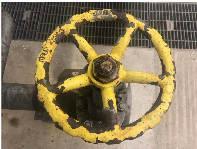
Figure 1. Partial corrosion and further expansion due to collision
