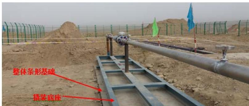
Figure 12. Schematic diagram of skid mount base
