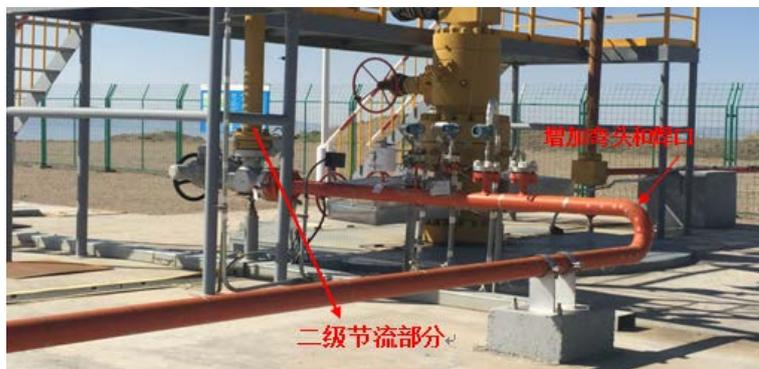
Figure 6. Schematic diagram of traditional single-well wellsite process pipeline
