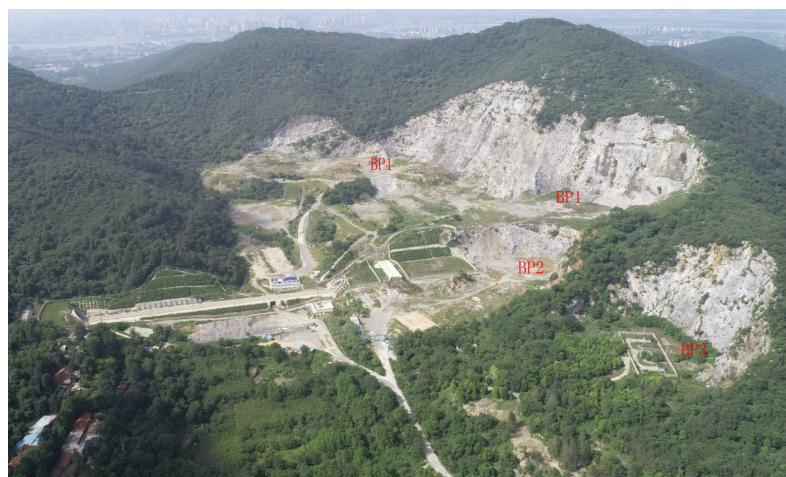
Figure 2. Present situation of mining slope in mining area
