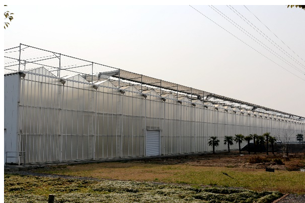
Figure 4. Dutch Venlo type greenhouse in Shanghai 图 4. 荷兰芬洛型玻璃温室(上海)
