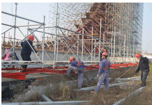
Figure 4. Construction site of ringlock steel pipe stent
