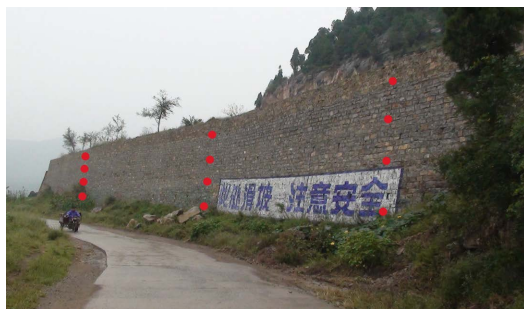
Figure 4. Layout of earth pressure monitoring points
