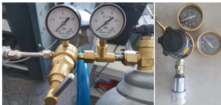
Figure 3. Pressure stabilizing valves at the outlet of gas tanks and chambers
