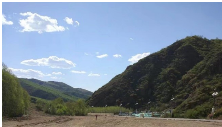
Figure 1. Construction site environment (Westward)
