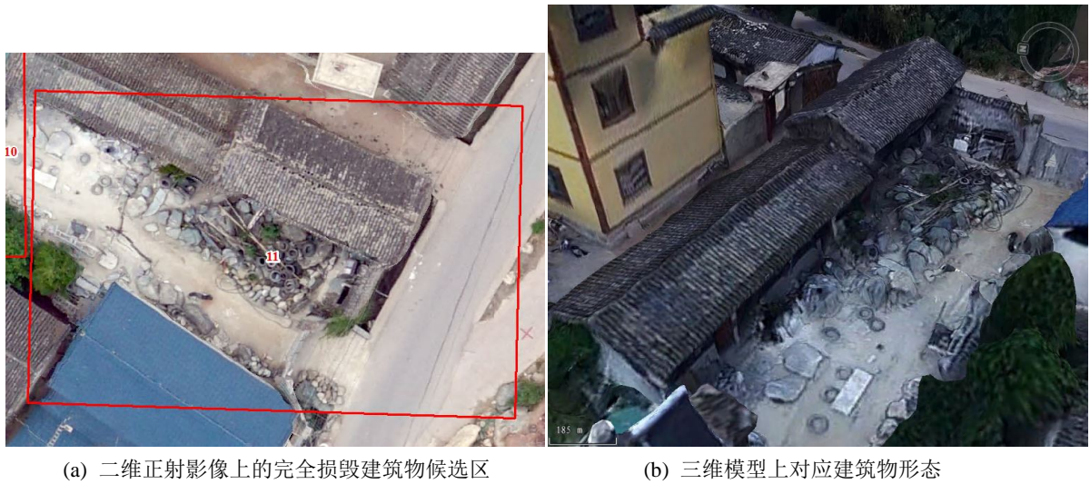
Figure 8. Candidate areas for completely destroyed buildings that are not easily identified by 2D orthophotos 图 8. 二维正射影像不易准确辨别的完全损毁建筑物候选区
