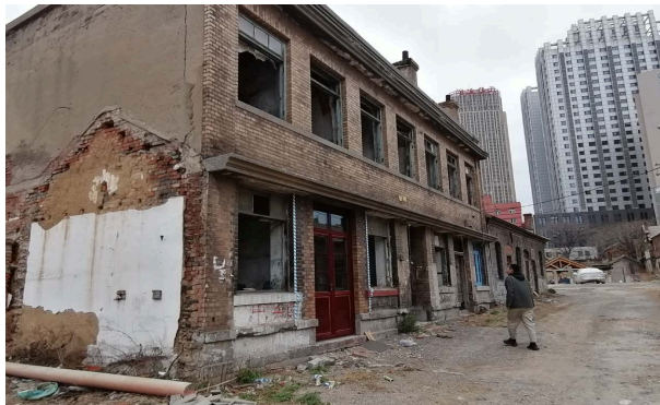
Figure 1. Dongguan street frontage shops 图 1. 东关街临街商铺
