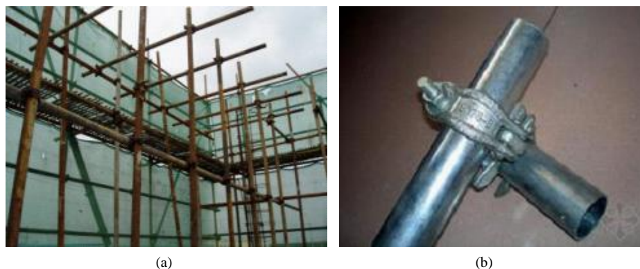
Figure 1. Steel tubular scaffold used in construction. (a) Complete picture; (b) Connected joints 图 1. 施工中采用的扣件式脚手架及节点。(a) 全景；(b) 连接节点
