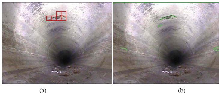
Figure 8. Recognition result, group (ii) (a) regional positioning recognition method; (b) Fracture feature search method
