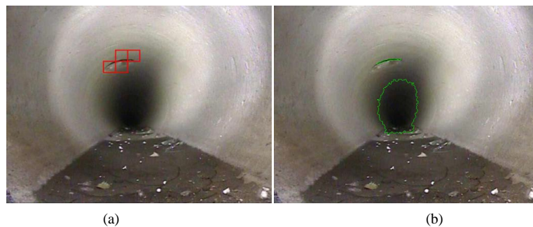
Figure 7. Recognition result, group (i) (a) regional positioning recognition method; (b) Fracture feature search method
