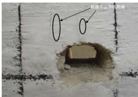
Figure 11. Upper crack of pressure relief roadway
