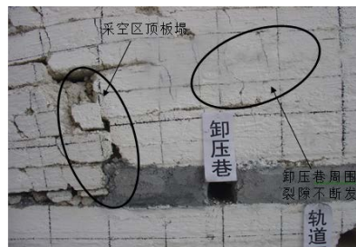
Figure 8. Cracks on top of goaf
