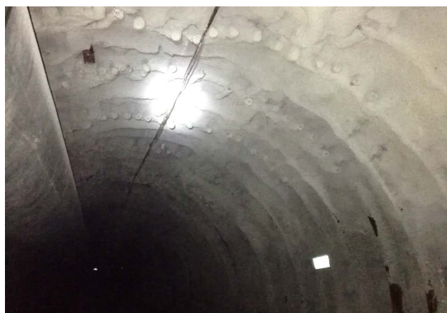
Figure 7. The effect of western third tape stone gate support 图 7. 西三胶带石门支护效果
