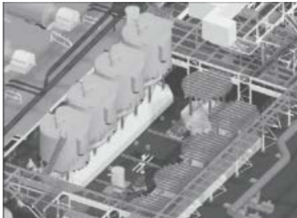
Figure 4. Removal of original steel structure and establishment of steel support on new foundation 图 4. 原有钢结构拆除及新地基上钢支撑完成建立
