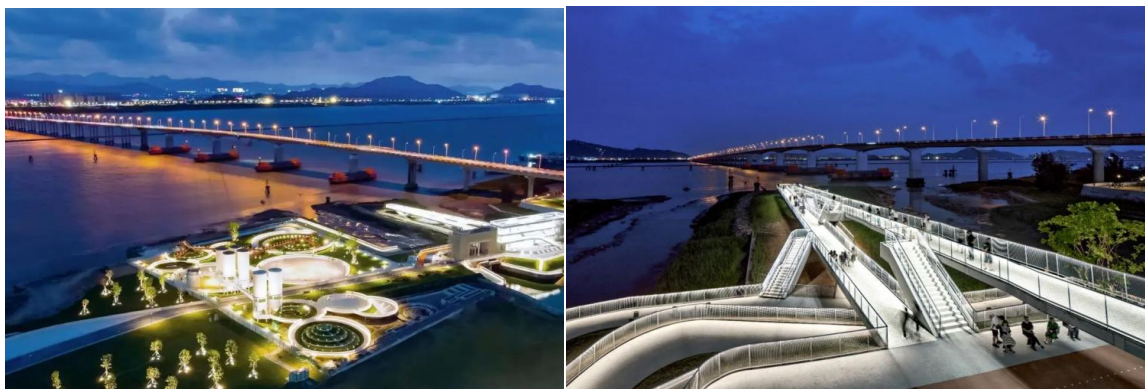
Figure 1. Taizhou Riverside public Space Demonstration project, as a demonstration section of riverside public space, has become a high-energy “light show” and a blunt steel channel
