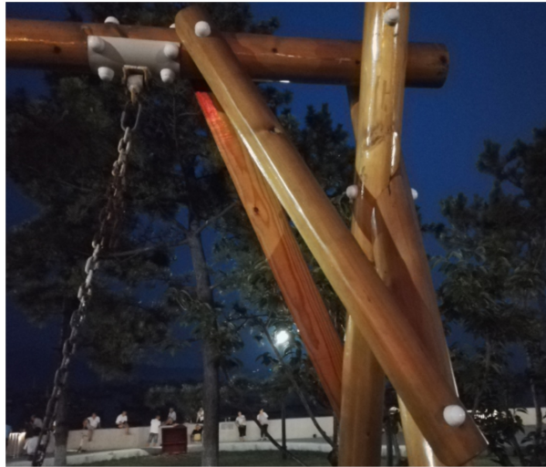
Figure 10. Corner strengthening rod of a certain swing 图 10. 某秋千的角部加强杆
