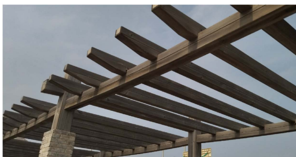
Figure 4. Wooden shed structure 图 4. 木质棚架结构
