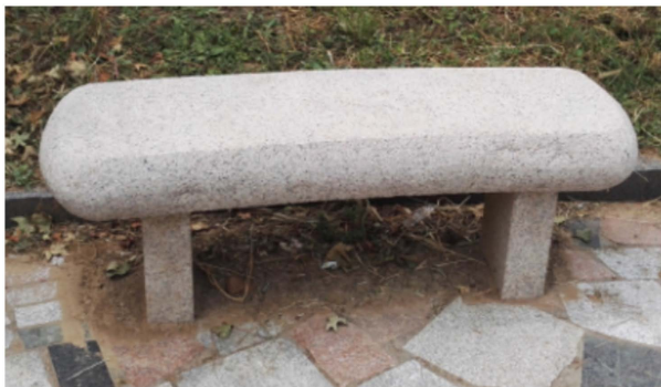
Figure 5. A simple supported stone bench with extended arms 图 5. 某伸臂简支石凳
